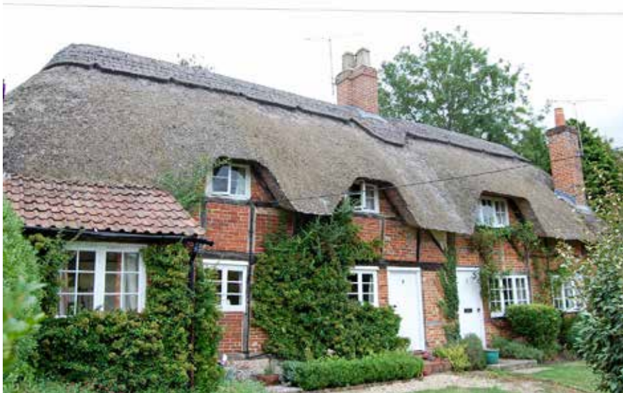
Figure 1. Nos 6 & 7 Mill Lane viewed from the north-west. The three eyebrow windows define the three bays of the house as originally built, but were almost certainly a later addition to provide lighting when the upper floors were inserted.
