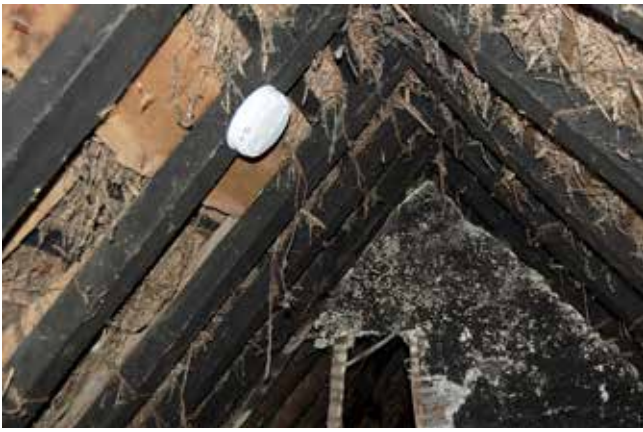
Figure 2. View of the upper section of the roof of the hall bay. Note the heavy sooting on the rafters, on the wattle and daub infill of the frame dividing hall and parlour, and even on some early thatching battens.
