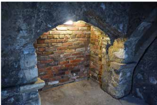
Figure 3 Crude eighteenth century fireplace inserted into rear of vault. (M. South)
