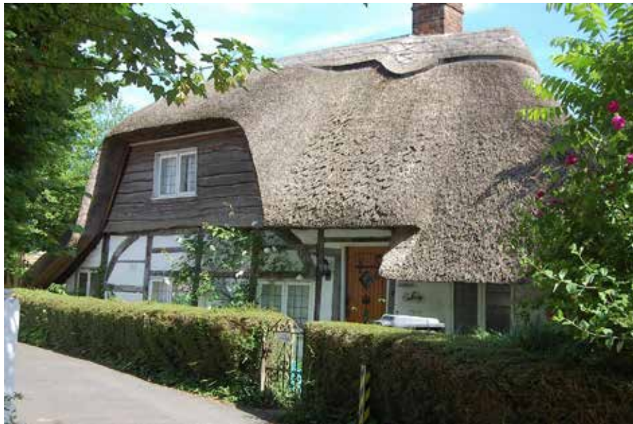
Fig.1. Tavern Cottage as it appears today. The roof dormer was the result of a later-20th century alteration to allow more headroom in the upper floor rooms.
