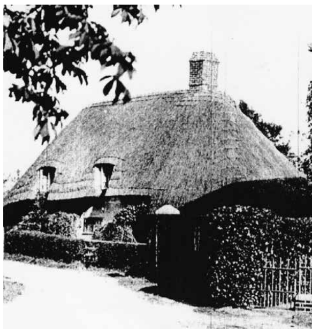
Fig.3. This photograph is from a postcard of 1909 and shows the roof before the later alteration. The two small eyebrow windows must have been at floor level in the upstairs bedrooms.
