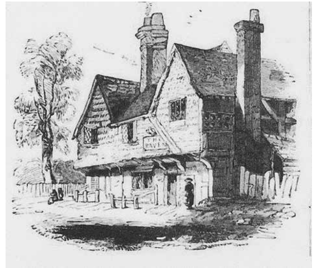
Fig.1. This 19th century engraving of The Raven shows the jettied south elevation viewed from London Road. The upper floor appears to be tile-hung, the tiles perhaps masking the poor condition of the framing which was subsequently restored soon after 1900 when it became a house.
