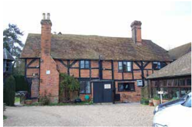
Fig.4. The eastern range exhibits a variety of infill brickwork. The incremental approach this illustrates is in contrast with the uniformity of the first floor of the restored southern range.
