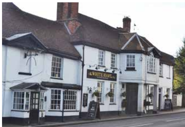
Fig.1 Contemporary photograph of the White Hart from the north. The 15 th century chamber range is the lower section of the building to the left. The taller right hand section appears to be an 18 th century rebuilding in the area where the open hall was located, and incorporates older timbers.
