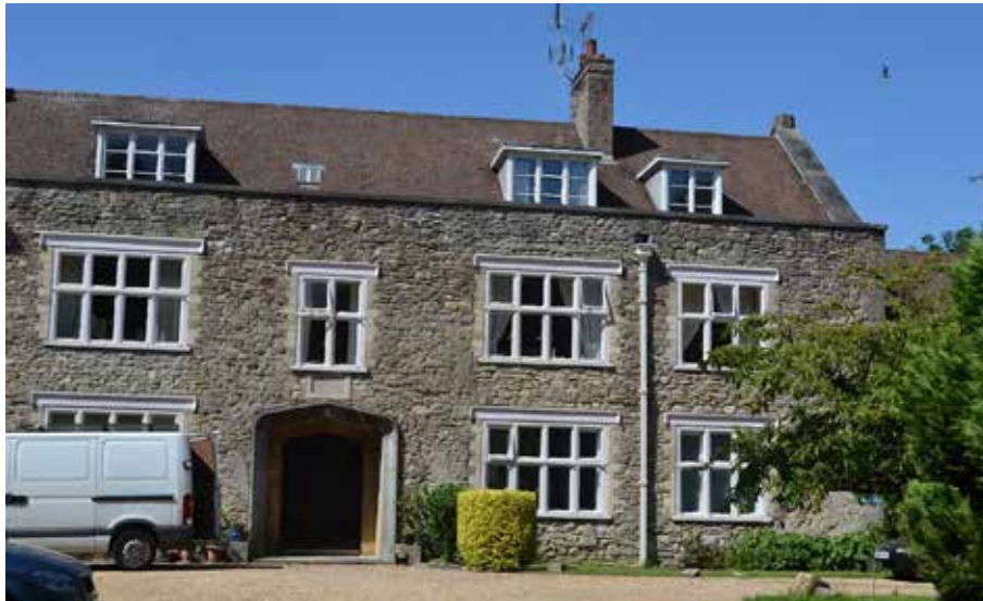
Bitterne manor house: some of the remains of the manor house were converted into a castellated country house, before being gutted by enemy bombing and subsequent conversion into flats
