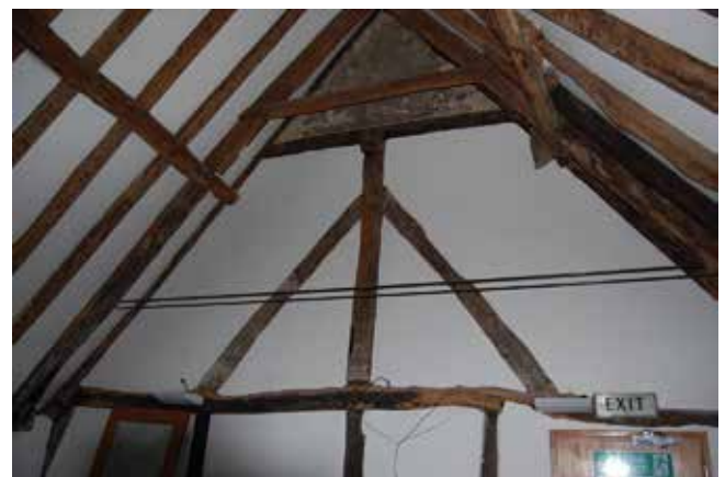
Fig. 1. The crown-post roof standing behind the present frontage of London Street (photo: Bill Fergie).
