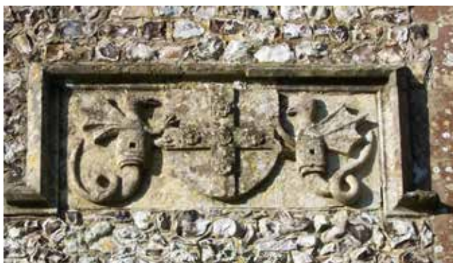
Fig. 3b. Langton's arm correctly positioned at the east end of East Meon Church where the bishops were rectors and thus responsible for the fabric of the chancel. Each dragon supporter is wrapped in a long barrel – a punning reference to 'lang tun'. (photo courtesy Michael Blakstad).
