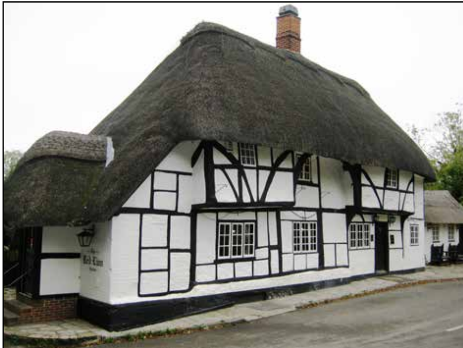
The Red Lion, Chalton. An original three bay Wealdon house, later added to at both ends
