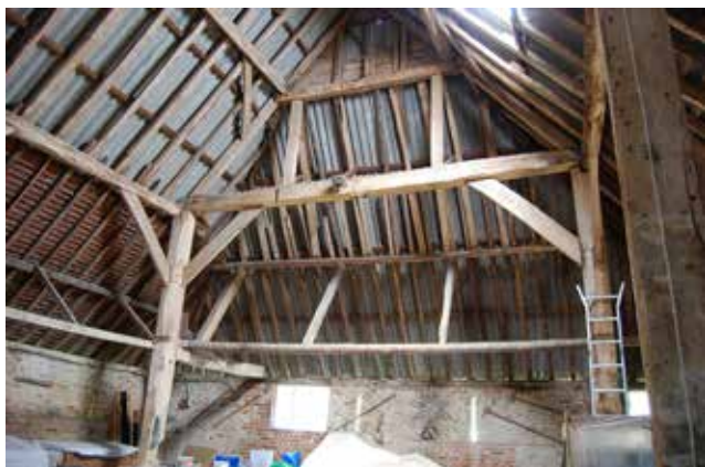
Fig.2. Interior view showing roof construction. (Bill Fergie)
