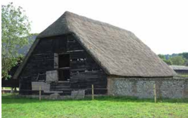
Fig. 2, building 1: A 4-bay thatched barn built in the late 17th century.
