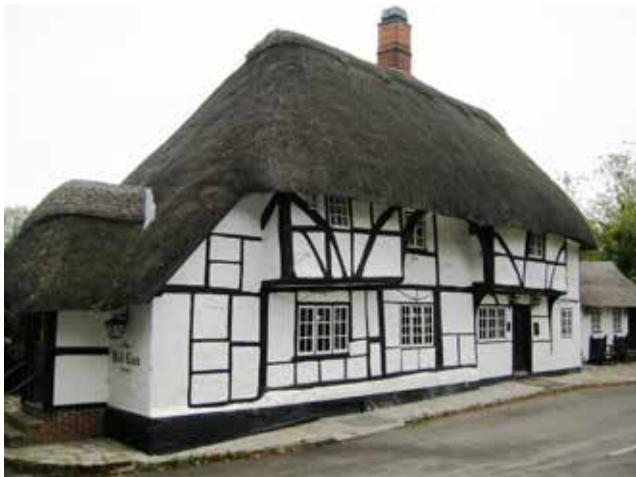
Fig. 1. The Red Lion, Chalton. The original three bay Wealden house was later added to at both ends.
