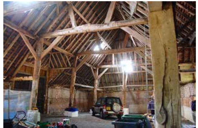
Fig.3. Interior view including evidence of bark on one of the main posts. (Bill Fergie)
