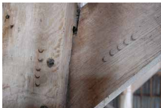
Fig.6. Carpenter's marks on adjoining timbers formed with a gouge. (Bill Fergie)
