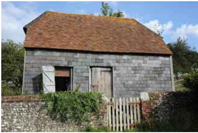
Fig. 4, building 7: A double staddle granary with slate walls, probably late 1850s.
