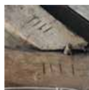
Fig.6. Carpenter's marks on adjoining timbers formed with a gouge. (Bill Fergie)
