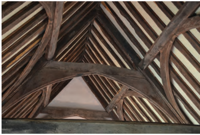
III: Newnham, the rebuilt roof from the second half of the fifteenth century
