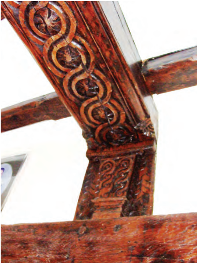
Fig. 4. Deane Cottage Sparsholt: part of the hall ceiling inserted in 1588-1620.
