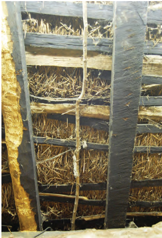
An unsoted hazel rod tied between sooted rafters at Silver Stream, Headbourne Worthy.
