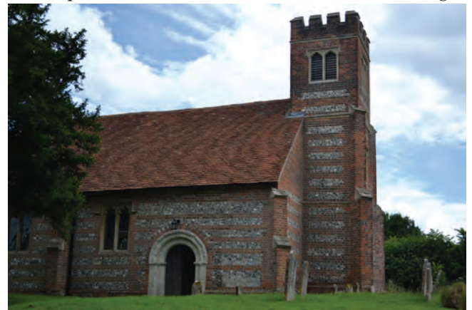
V: Up Nately showing the elaborate twelfth century doorway, the refaced brick and flint walls and the new tower of 1844
