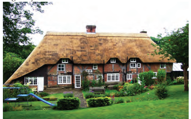
Fig. 3. Deane Cottage, Sparsholt, 1498.
