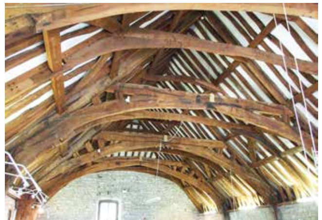
Fig 1: The Wool House, Roof
