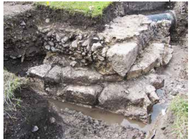
Figure 2 – St Elizabeth's College, Winchester. Foundations at the NW corner of the church. Three phases of building activity can be seen.
