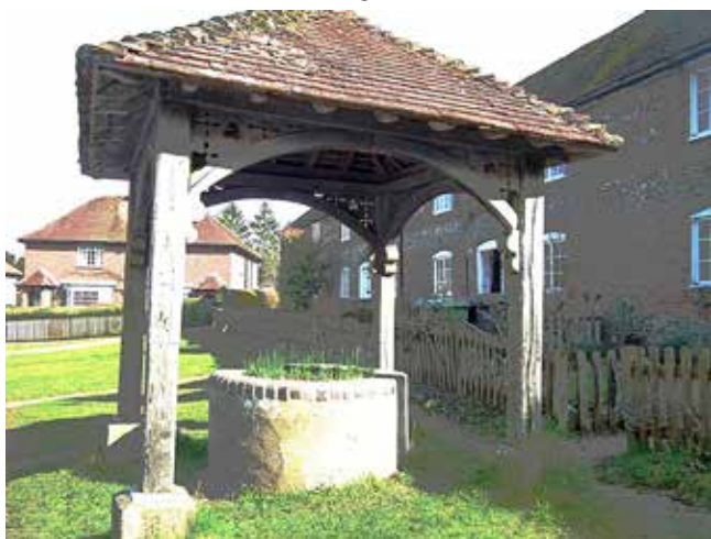
Fig. 2. Avington wellhouse and the cottages it served.
