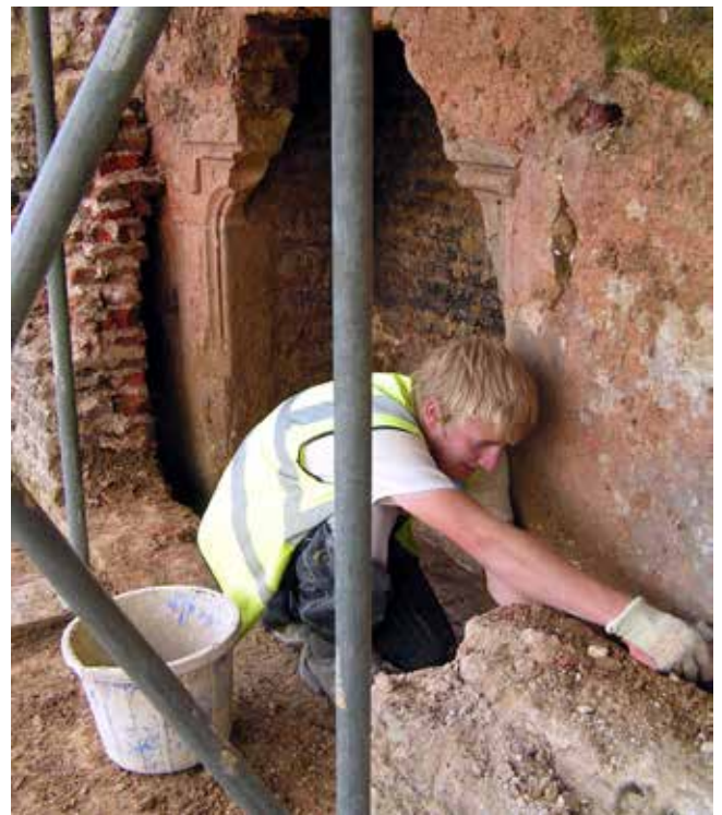
Fig 5: Dave Phillips, one of the workmen, tidies the fireplace surrounds
