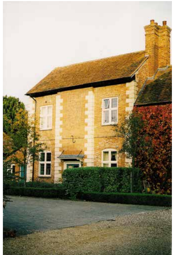
" Figure 3. James Zouch's brick-built tower, with raised and plastered-over brick quoins; presumably in imitation of the more expensive stone quoins of the earlier buildings at Place House. The original upper storey has been truncated"
