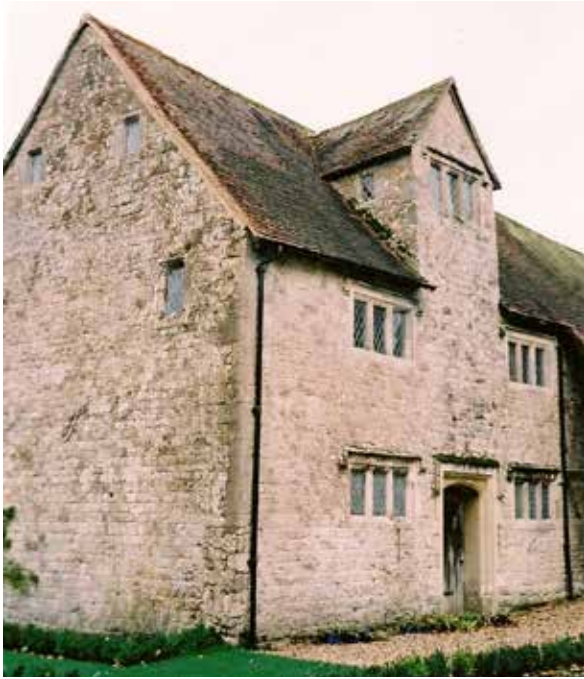
Fig. 2. The south-west corner of the stables showing the mid-17th-century windows with hood moulds. (photo – Jane Hurst)
