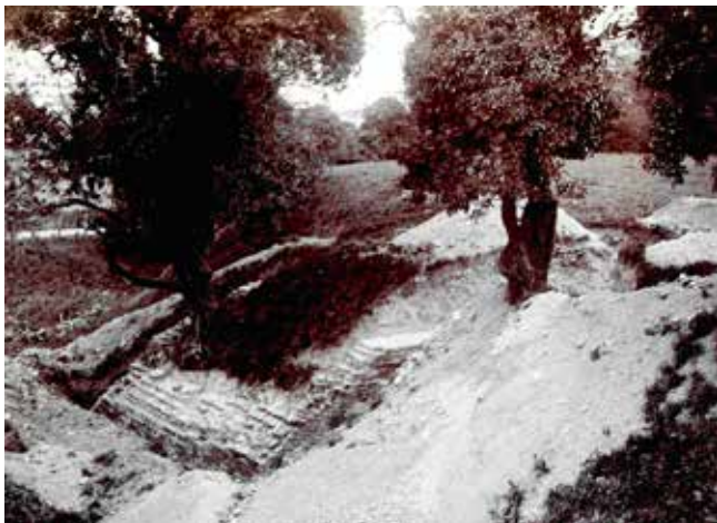
Figs 1 and 2 Excavations 2009 and 1904 from the same vantage point
