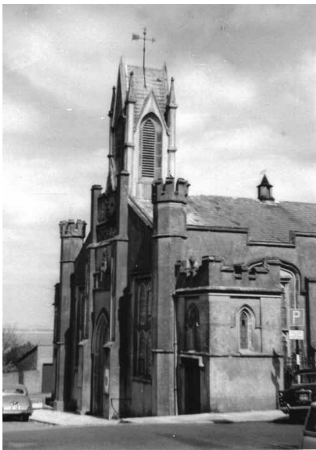
RYDE – The church of St. James, Lind Street. Built as a proprietary chapel in 1827 from the design of Greenway Robins of Walworth, London. The exterior before removal of details in the restoration of 1968-9. (Photograph: Rodney Hubbuck).
