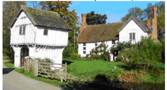
Fig. 5 Lower Brockhampton Manor House.
