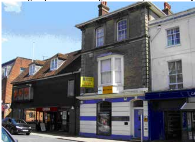
Fig.3 Shops occupying the former front of The George, a medieval inn.
