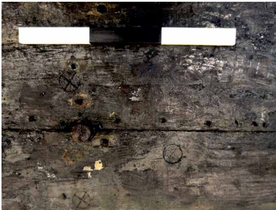
Fig. 5 Detail of wedged treenails and square shafted iron nail holes
