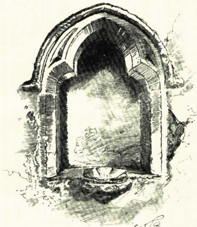
Boldre Church. Hants. Piscina in Tower
