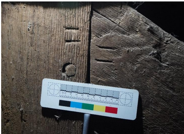
Fig 4. Tower. Bell chamber. Joint marked II
