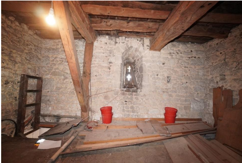
Fig 1. Church tower. Second floor
