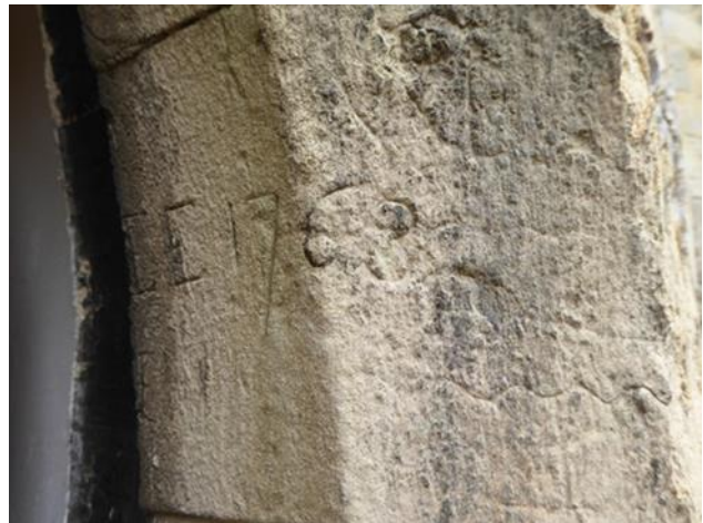
Fig 17. Tower. West doorway. South jamb. IE 1763. VV above
