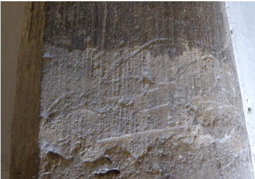
Fig 27. South nave. Pilaster. Curved lines
