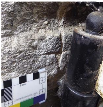
Figs 23 & 24. South doorway. East jamb. Crosses
