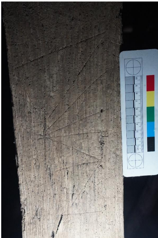
Fig 6. Tower. Bell chamber. Bay 1. Carpenter's marks
