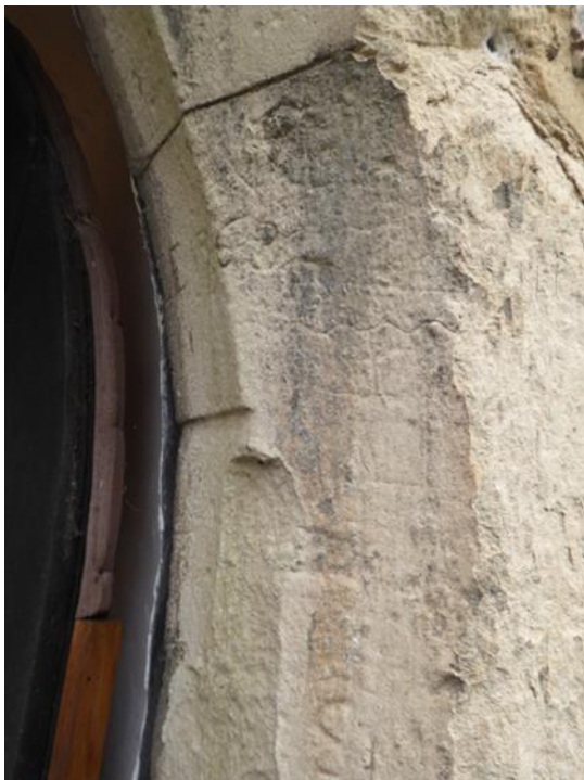
Fig 18. Tower, West doorway. South jamb. Initial S
