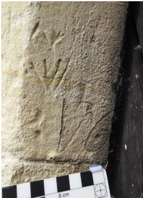
Fig 16. Tower. West doorway. North jamb. Partial date 176 with VV above
