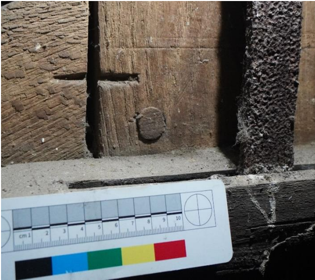
Fig 5. Tower. Bell chamber. Joint marked I
