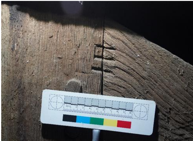
Fig 3. Tower. Bell chamber. Joint marked III
