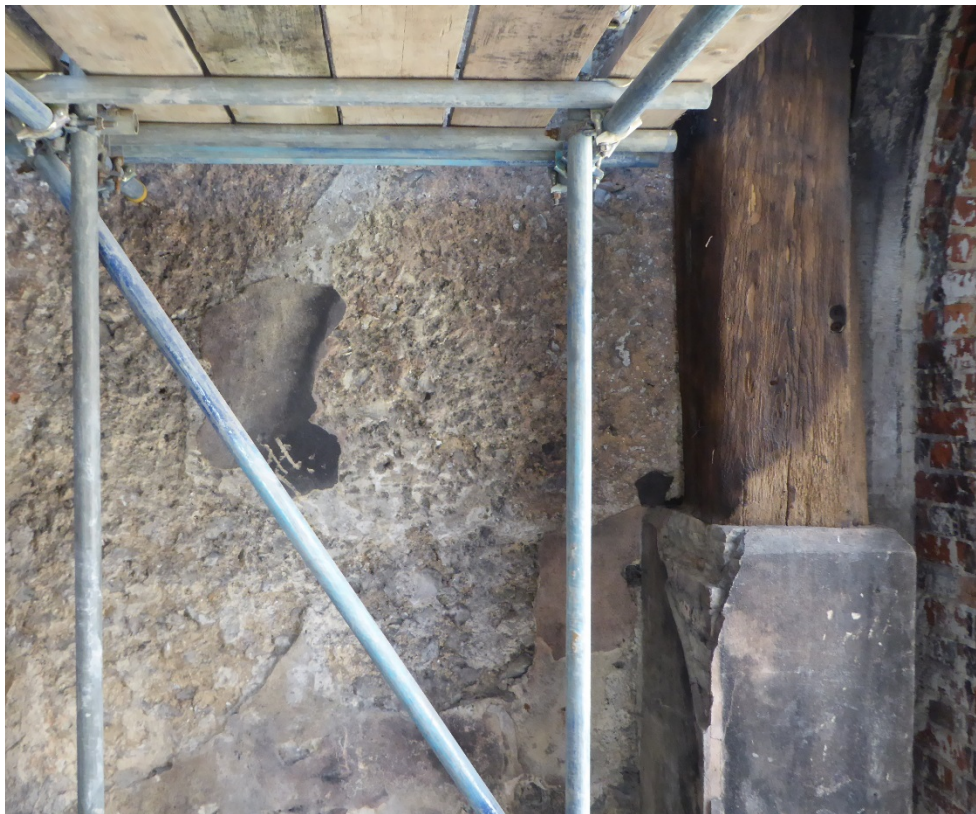
Figure 4 Location of plaster with consecration cross inside tower
