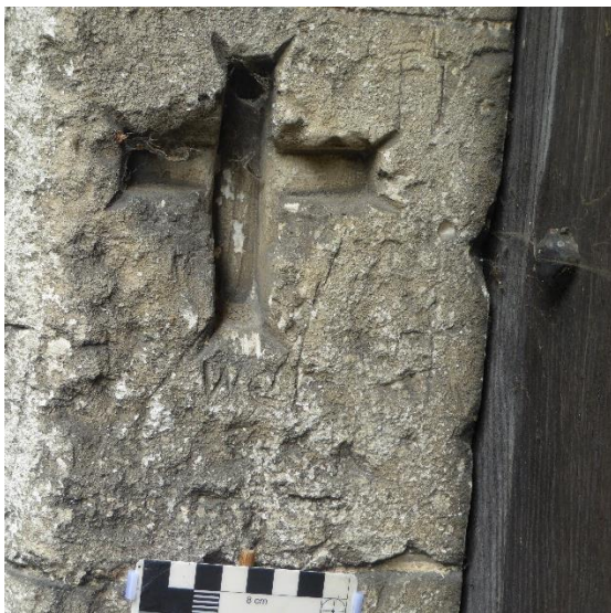
9 Deeply gouged cross shape, north side of door
