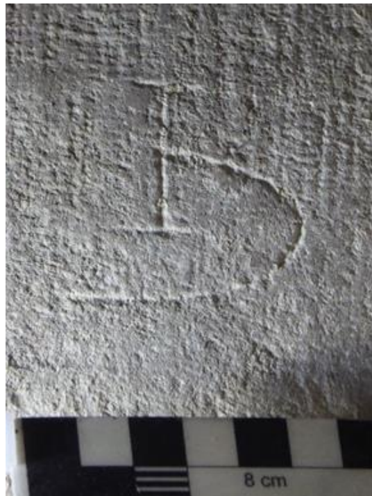
25 Tower arch, south side, mason's mark
