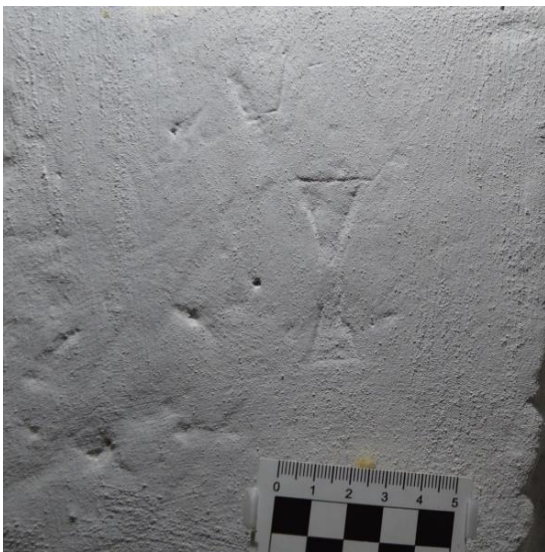
24 Ringing room, south window, possible mason's mark
