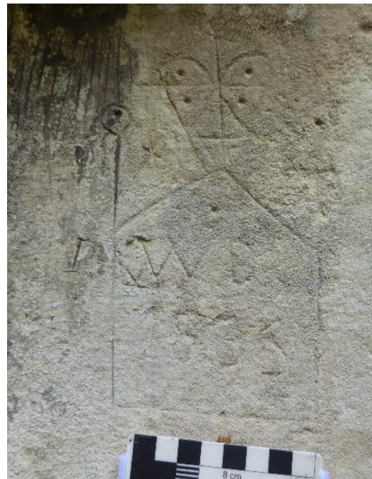
3 South side of doorway, WB 1833
