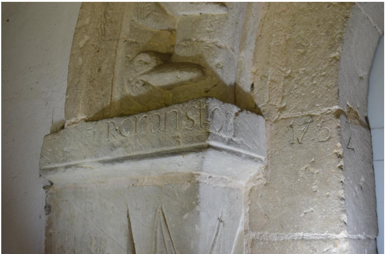
7 South doorway, west side. R. Cranston 1752 inscription running around impost onto arch
