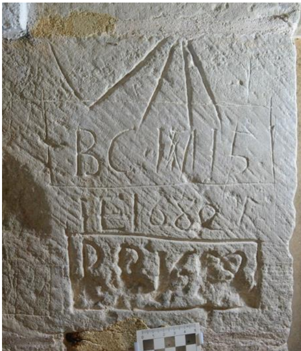
5 South doorway, west side. Boxed sets of initials from the 1600s and 1700s. Scratch dial at top of block
