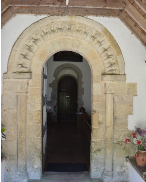
1 The south doorway with beakheads
