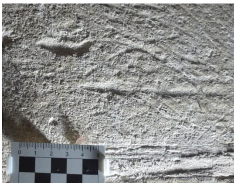
9 South doorway, west side. Possible mason's mark
