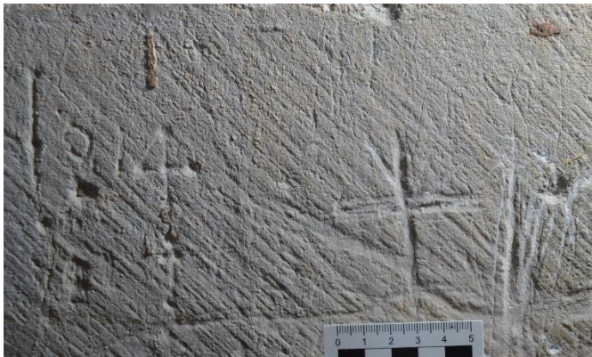
11 Chancel arch, north jamb, crosses
