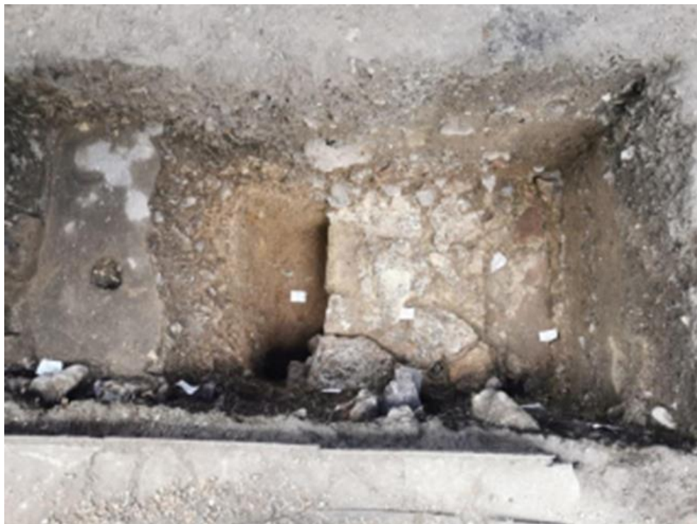
Fig 18 Hyde900: concrete slab associated with the Anderson shelter alongside the Abbey wall foundation and robber trench
