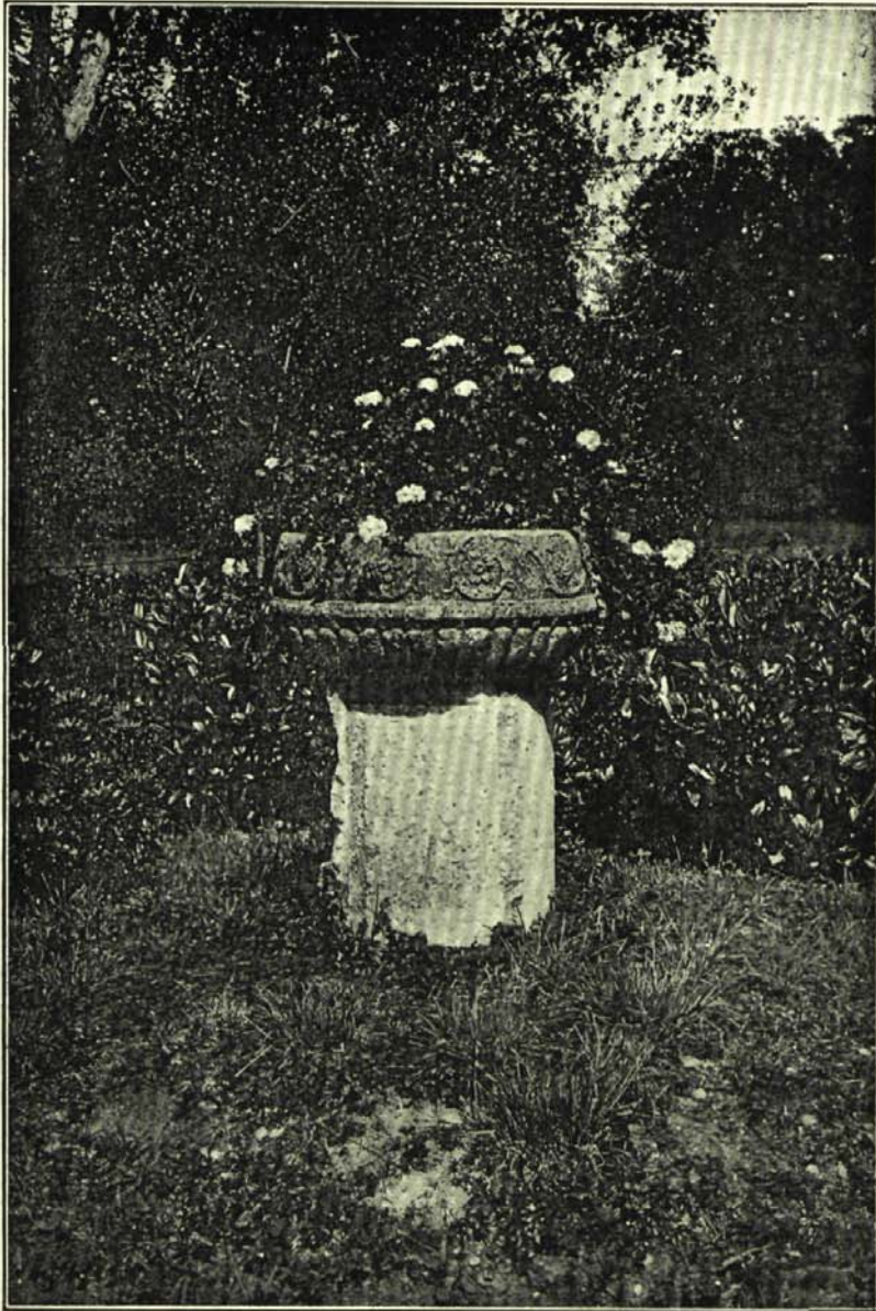
REMAINS OF THE OLD MANSION AT FARLEY, NOW AT THE RECTORY.
