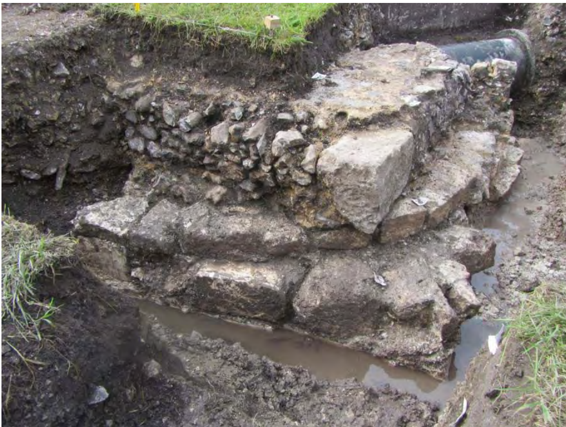
Fig. 11 St Elizabeth's College, Winchester. Foundations at the NW corner of the church. Three phases of building activity can be seen
